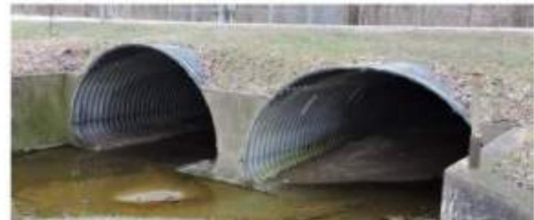
Proposed culverts improve fish habitat, can be visually inspected, and are large enough to accommodate tidal fluctuations and heavy rainfall.
