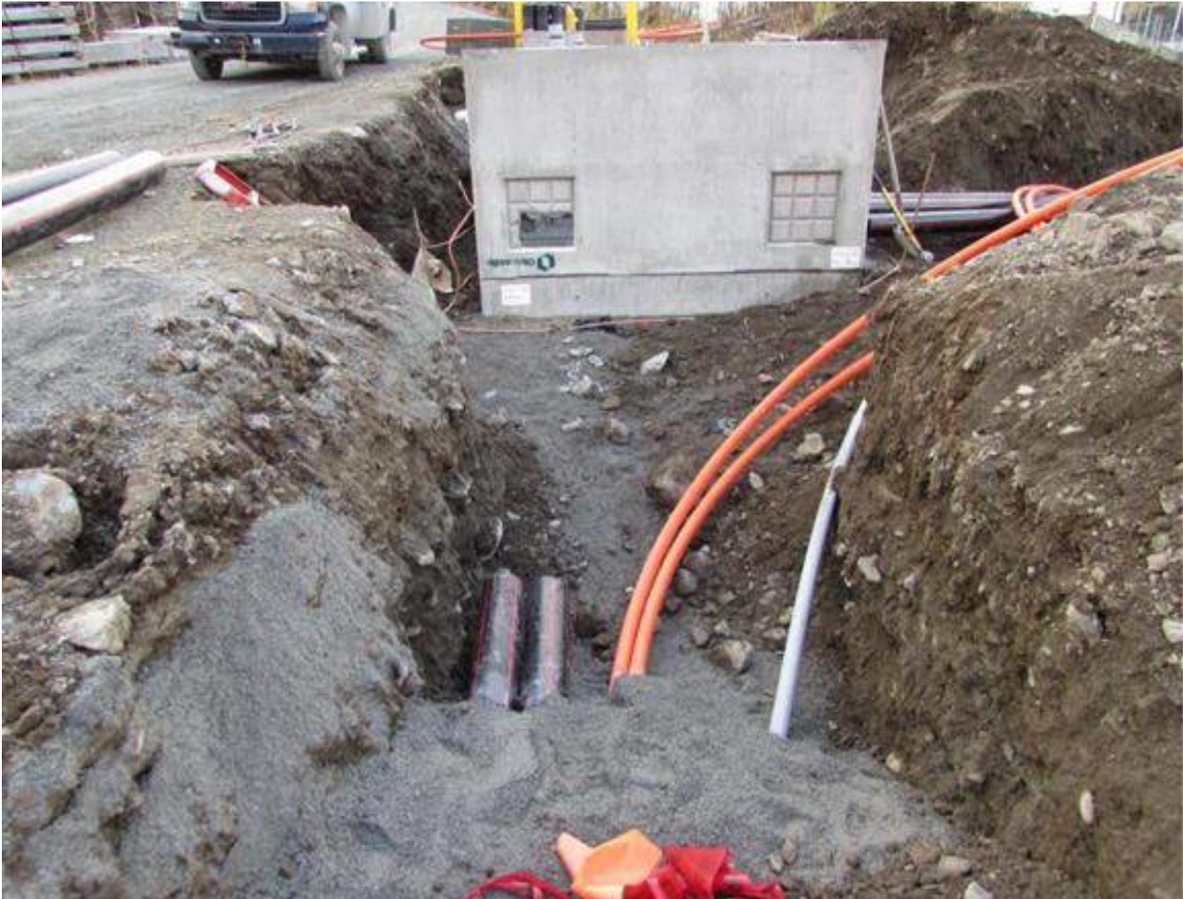
Fiber optic cable is typically laid in 2" orange conduit.
