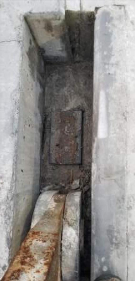
Crane Tie-Down Vault with no drain.
