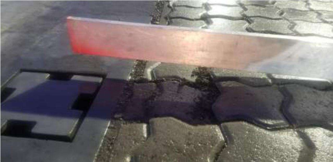
Paver blocks exceed allowable height tolerance
