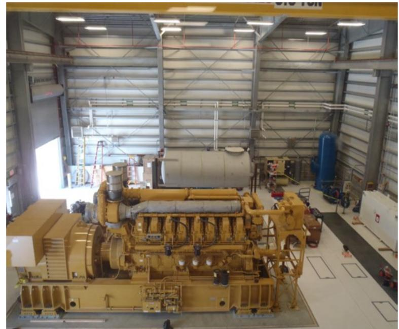
**PROJECT DESCRIPTION:** This project consists of the inspection, major maintenance, and rebuilds of the primary Generator sets in the Unalaska Powerhouse. The maintenance schedule for the generator sets at the Unalaska Powerhouse is determined by engine hours. Engine inspections are also conducted by manufacturers mechanics to determine if engine rebuilds are needed according to the hourly schedule or can be prolonged.
