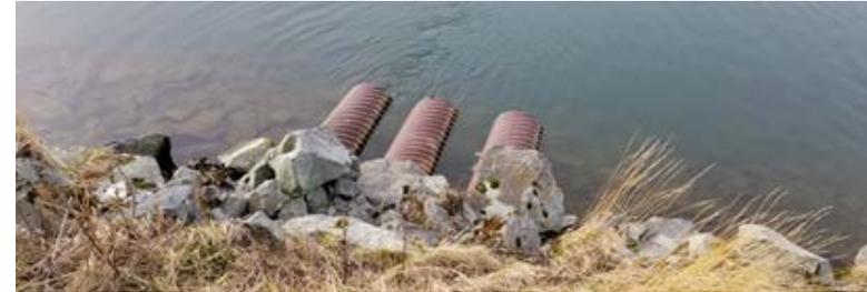
Existing Culverts are Failing
